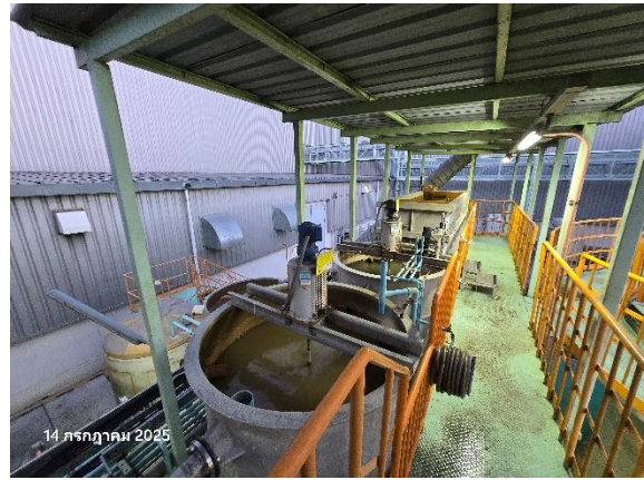
Coolant Wastewater Treatment System
