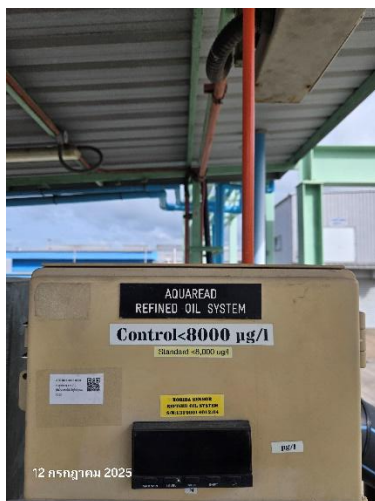
Oil & Grease Meter UT2
